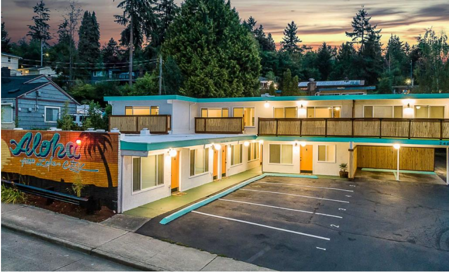
Aloha house - 10 unit mid-century apartment building in Lake City. Full studs out renovation.
