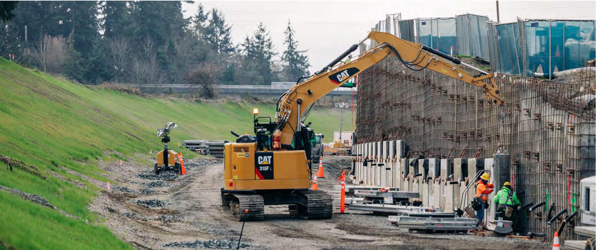
Construction of retaining wall for Federal Way Link Extension
