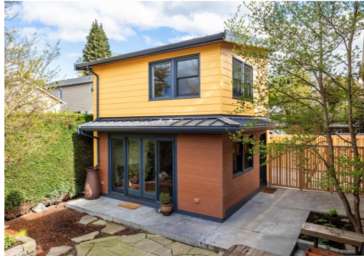
A detached ADU (DADU) , sometimes called a backyard cottage, is an ADU in a separate accessory structure.
