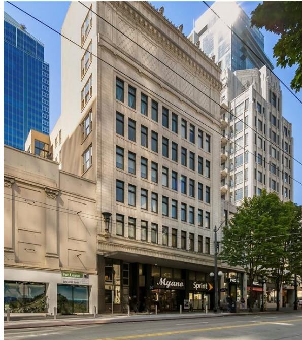
Figure 12 Picture of the Fisher Studio Building
