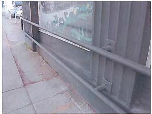
Detail, east elevation, showing corner and mid-elevation fluted pilasters. The railings were installed some time after 1966.
