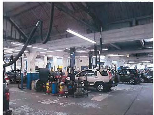
Interior, second floor automobile service area, showing concrete beams and wood roof trusses
