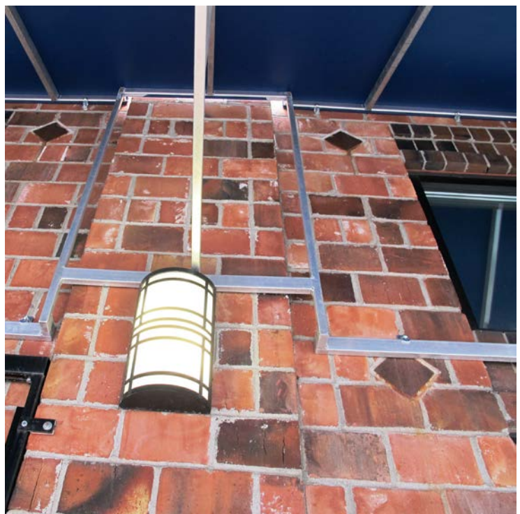
Detail, west elevation (facing First Avenue S.). Diamond-shaped tiles, shaped window headers, windows, and light fixture are non-original and date from a 2003 renovation. Compare to 1937 tax assessor photo.
