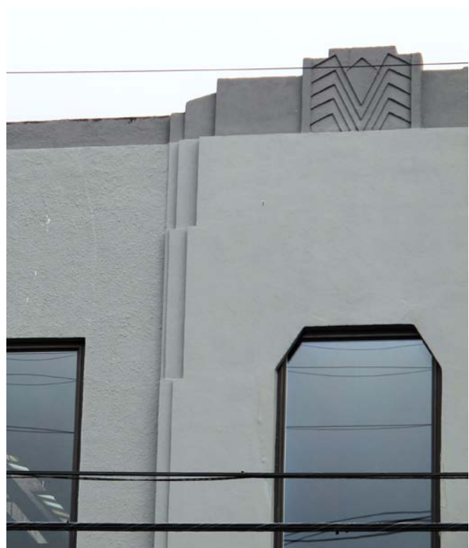
Detail, west elevation (facing First Avenue S.), and exterior finishes. All windows on this elevation are non-original.
