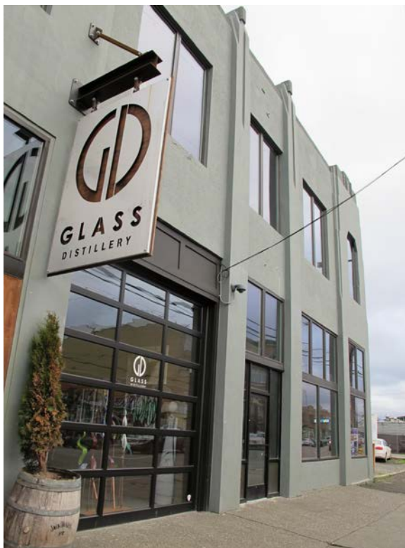
Detail, west elevation (facing First Avenue S.), and exterior finishes. All windows on this elevation are non-original.
