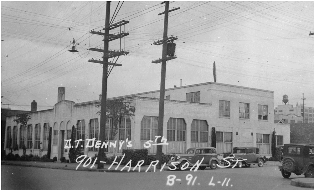
Pioneer Sand and Gravel Company Building, 901 Harrison Street, c. 1937
