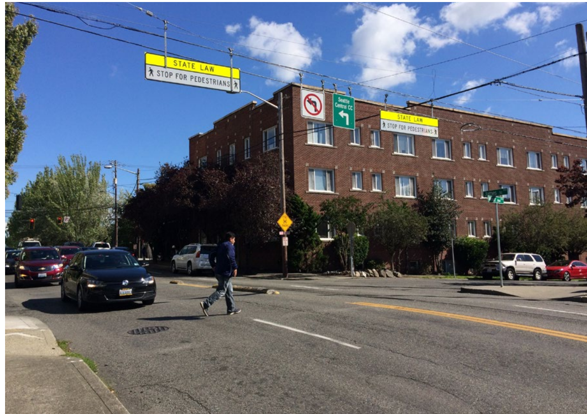
Minor and James Crossing Existing condition looking east
