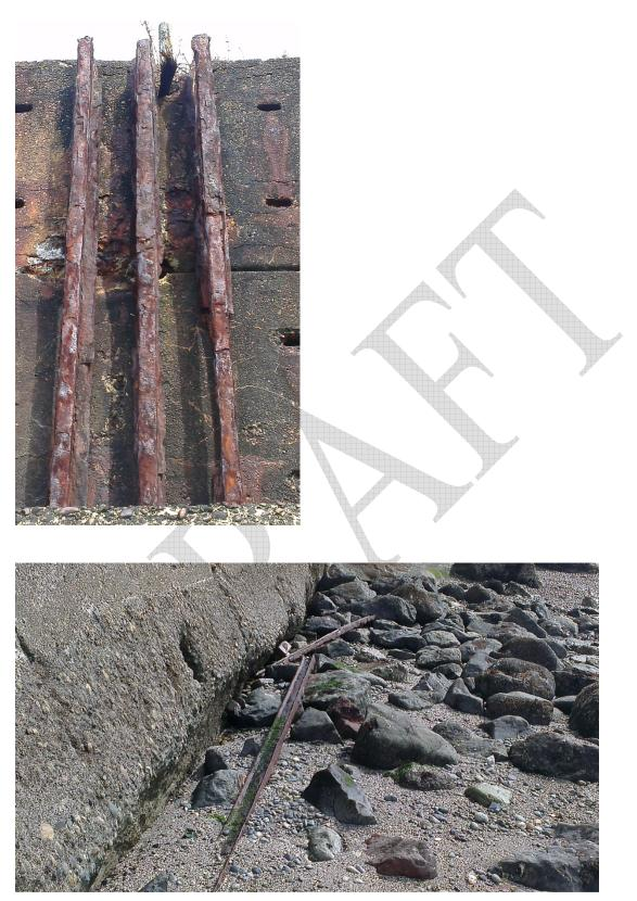
Figure 3. Corroded steel rails and failed top waler which historically held tie back anchors. Also note scour of sediments adjacent to concrete footing.
