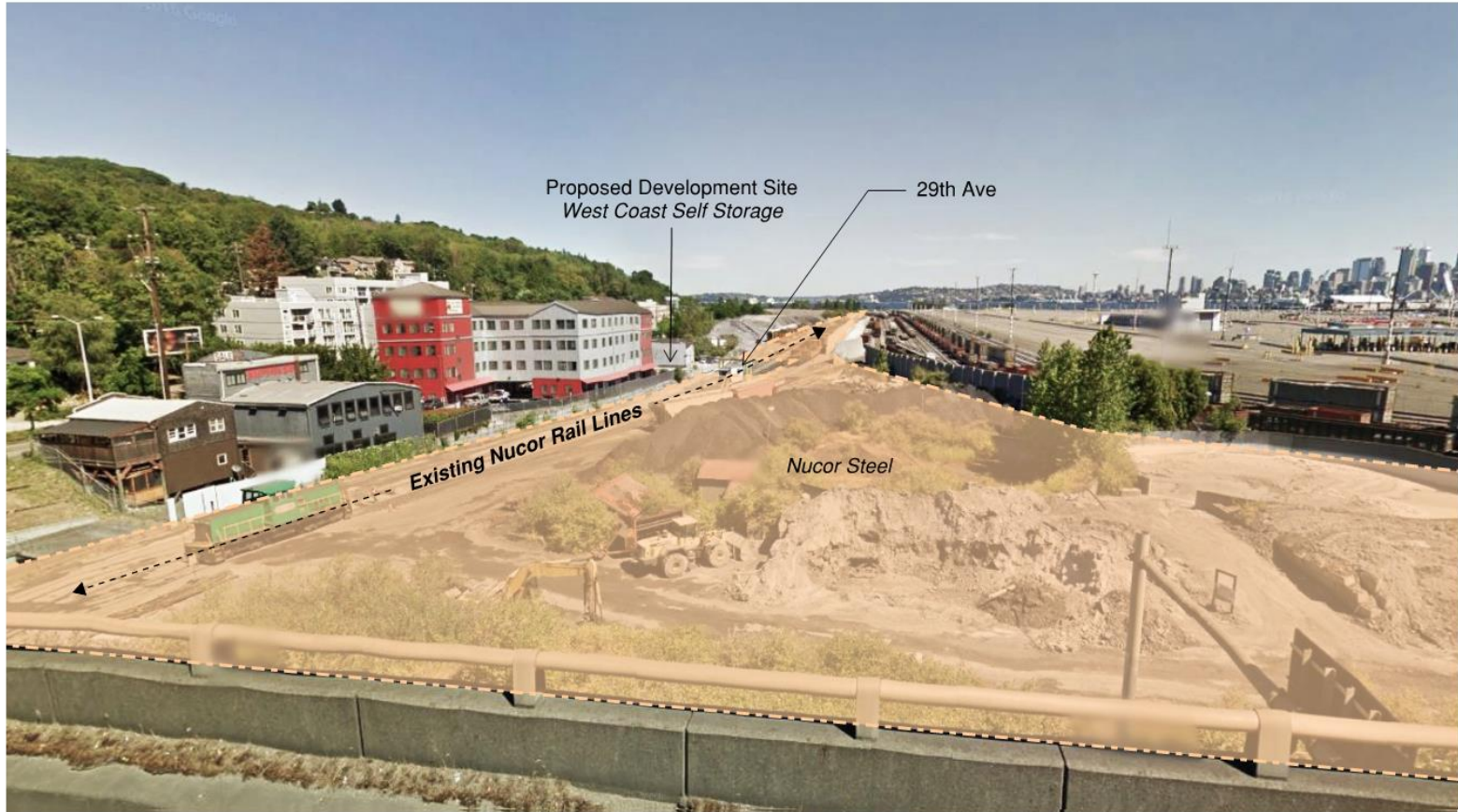
Nucor Rail Lines from West Seattle Bridge
