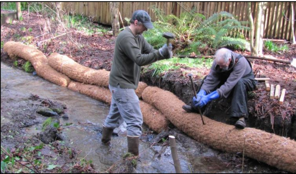
Steve Winter and Mark Harmon secure coir logs to stabilize and rebuild the bank.
