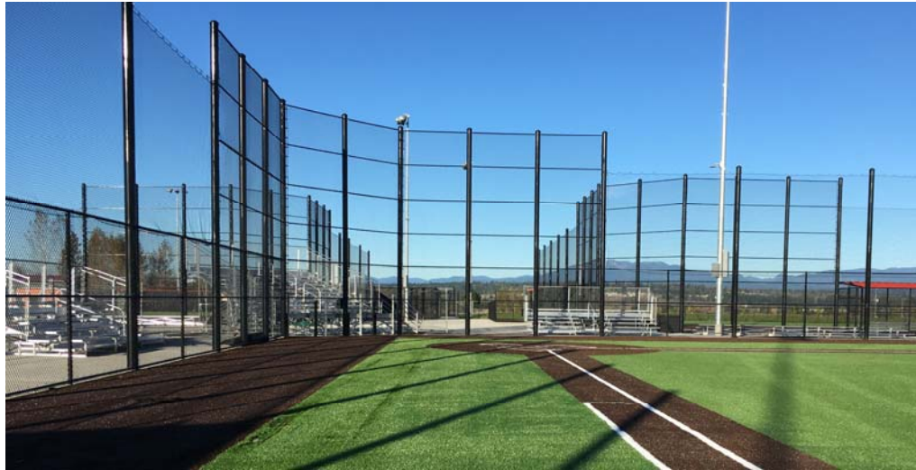
Example Baseball Backstop, note – in this photo there is a duplicate backstop to the right and beyond.
