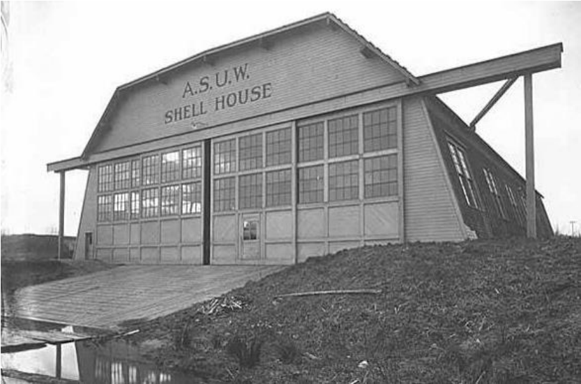
UW Canoe House/ASUW Shell House, 3655 Walla Walla Road NE, 1923
