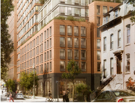
Transition to the adjacent townhouses.
