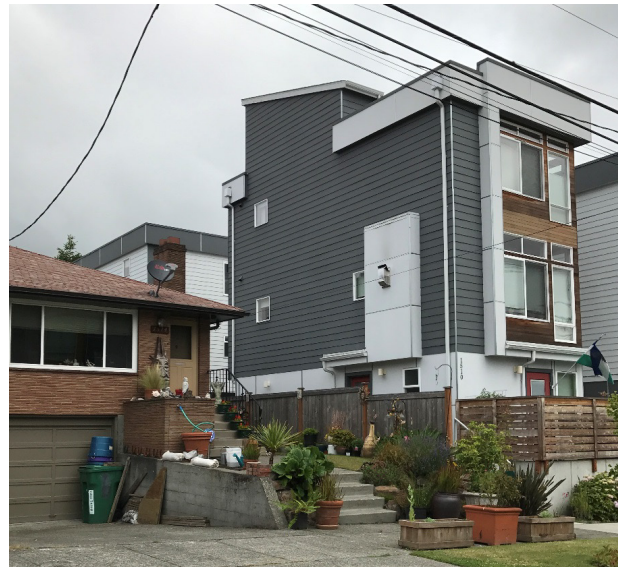
New side facade standards in the LR zone would prevent unfriendly blank facades at the edges of infill developments, like the condition shown here.
