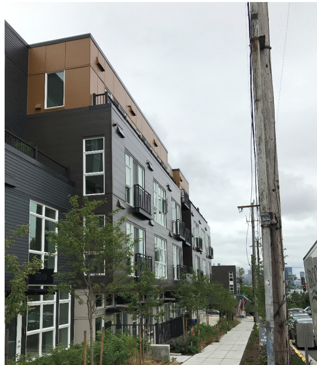
Street facing upper level setback standards in commercial zones would mitigate additional bulk and scale of taller buildings as seen from the sidewalk.
