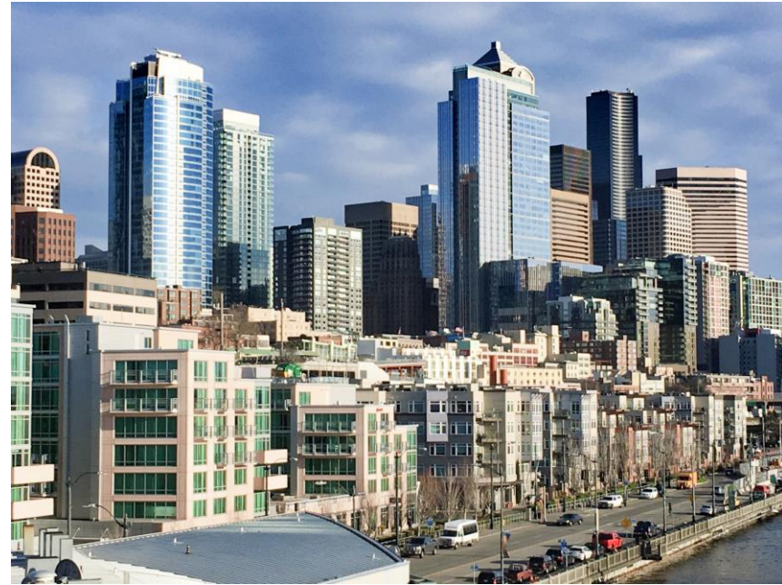
Tower designs contribute to the skyline
