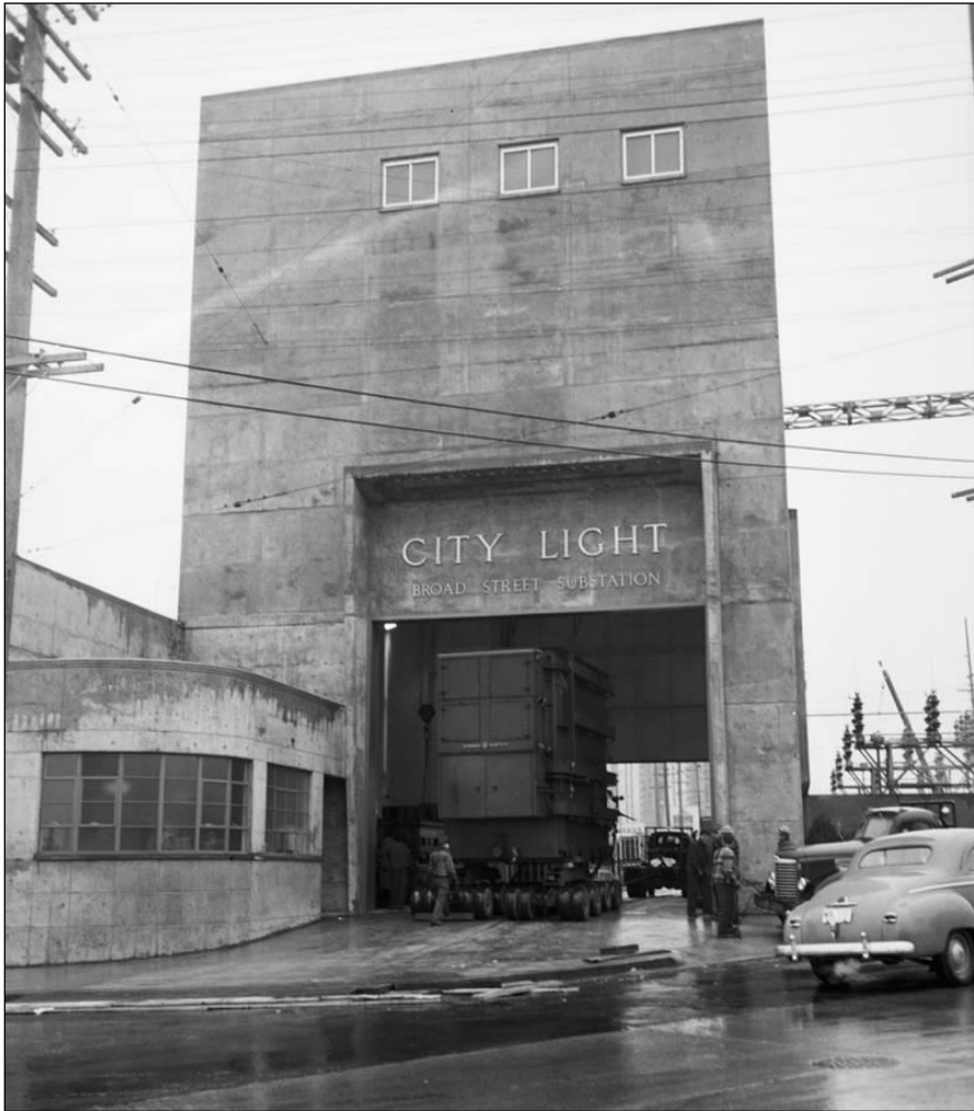
Broad Street Substation, 319 6 th Avenue North, 1950
