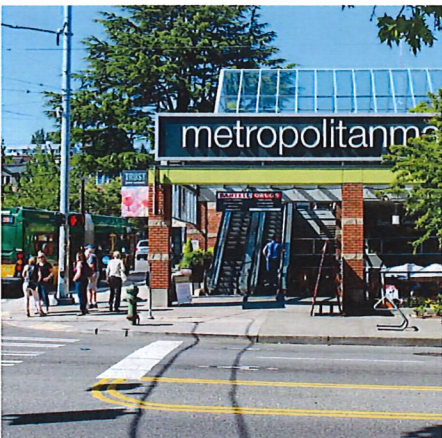
A corner setback and escalator help activate and connect the Heart of Uptown.
