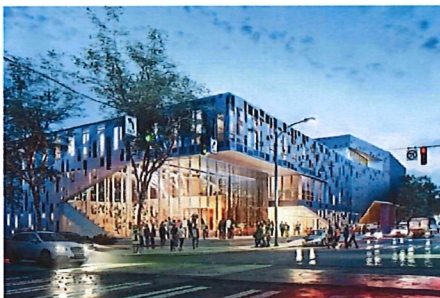
Creative treatment of the building facade and lighting make the arts visible to passersby.
