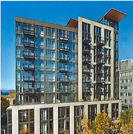
Modulation with contrasting color creates visual interest when viewed from a distance.
