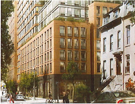
Transition to the adjacent townhouses.
