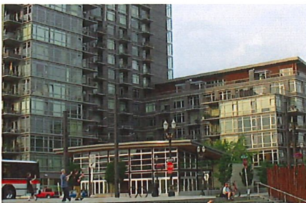
Taller building form is sited and oriented to minimize shadows on the open space.
