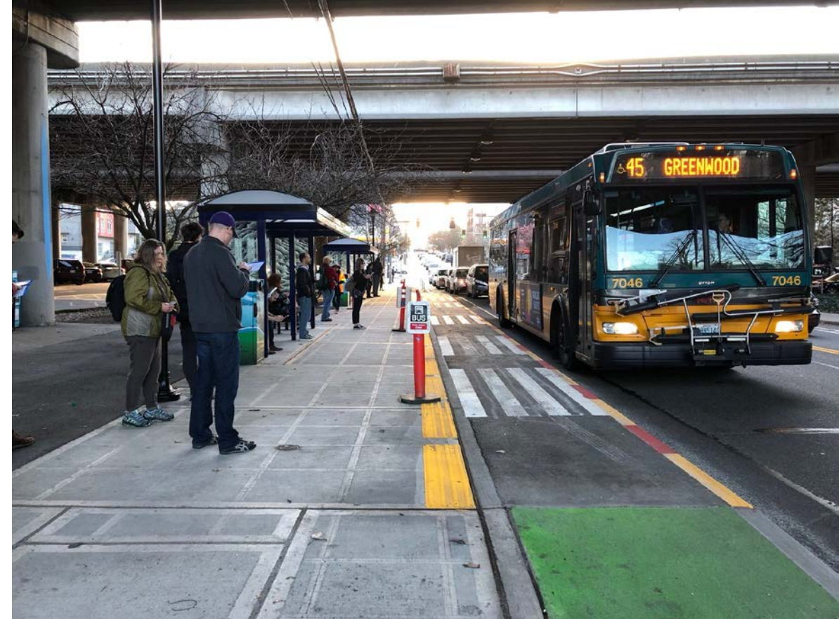
The completed NE 65th St Vision Zero project and protected bike lane
