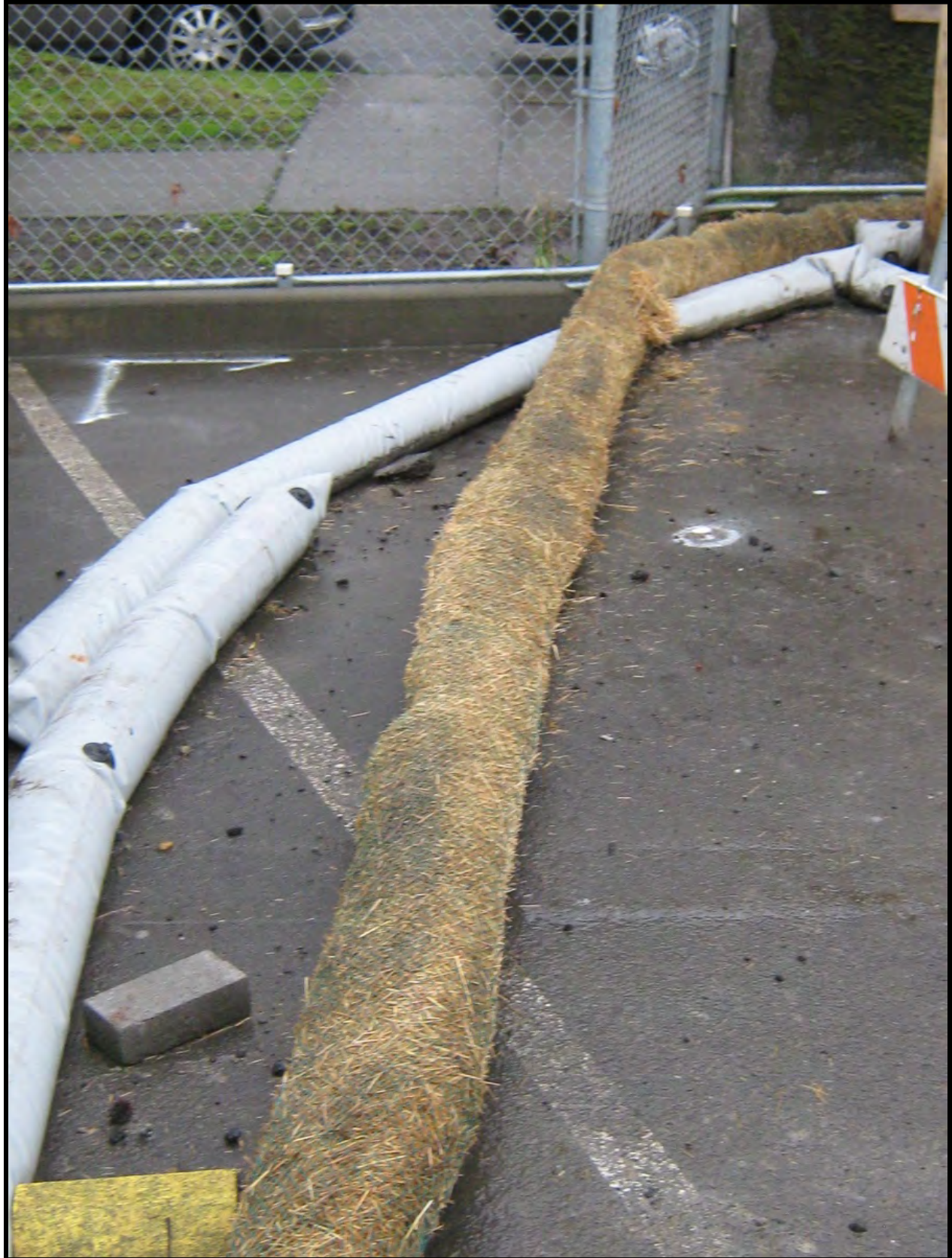
Figure 16. Curb and Gutter Barrier.
