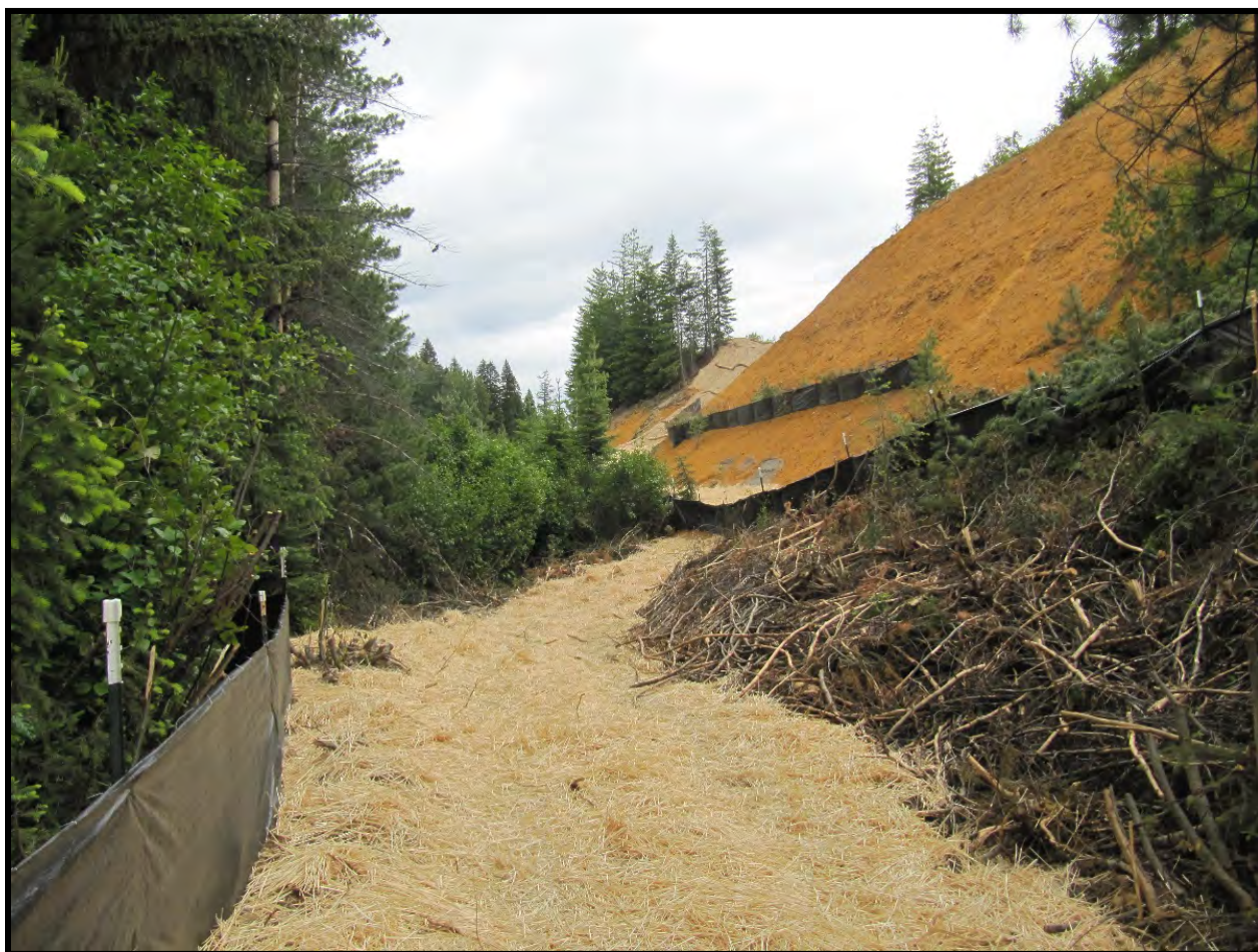
Figure 13. Filter Fence Installed on a Slope.
