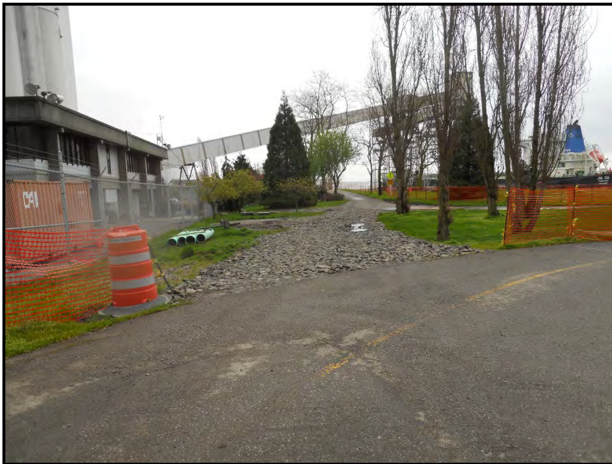
Figure 7. Stabilized Construction Entrance Access .
