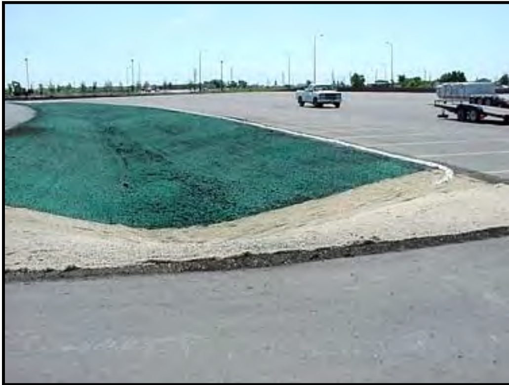
Figure 1. Hydroseeding Method.
