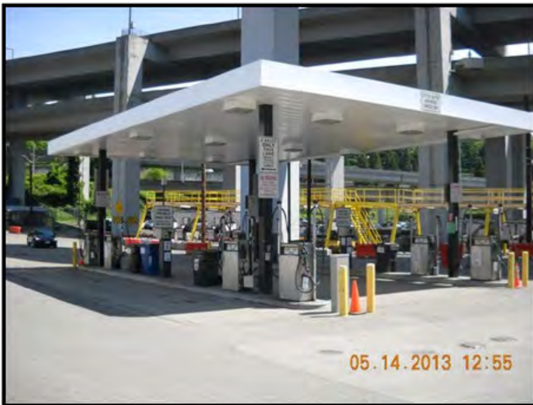
Figure 48. Roof at Fueling Island to Prevent Stormwater Run-On.
