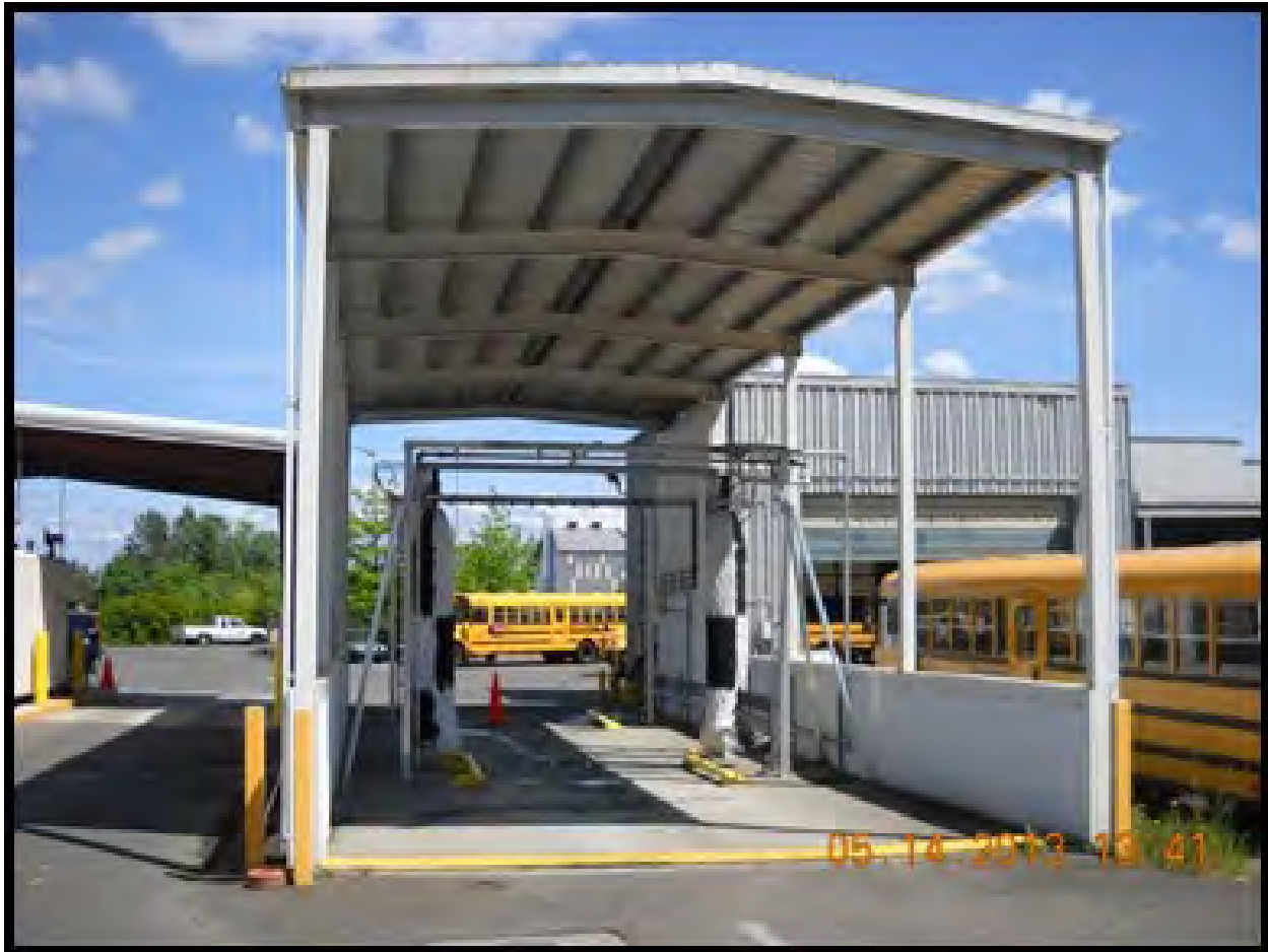
Figure 6. Car Wash Building with Drain to the Sanitary Sewer.
