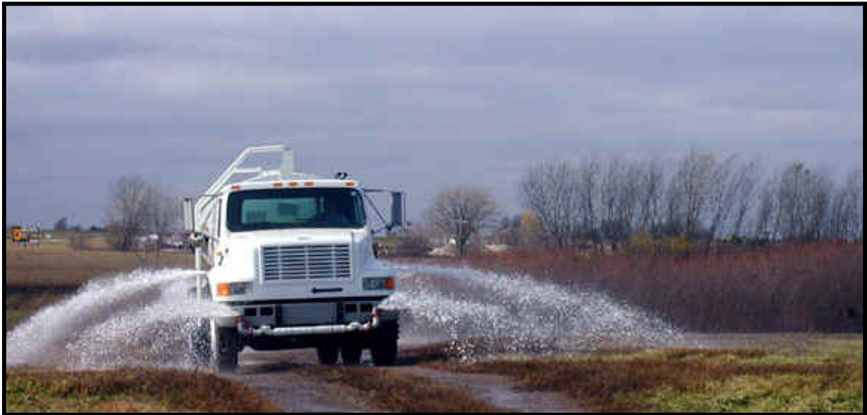
Figure 11. Using a Water Truck for Dust Control.
