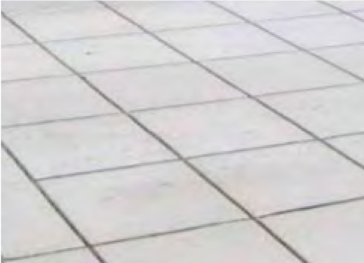
1: SDOT Standard Concrete 2'X2' scoring and sawcut joint
