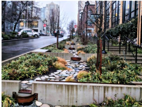
Figure 6: A stormwater project runs along Vine Street downtown. Photo credit: SDOT.
