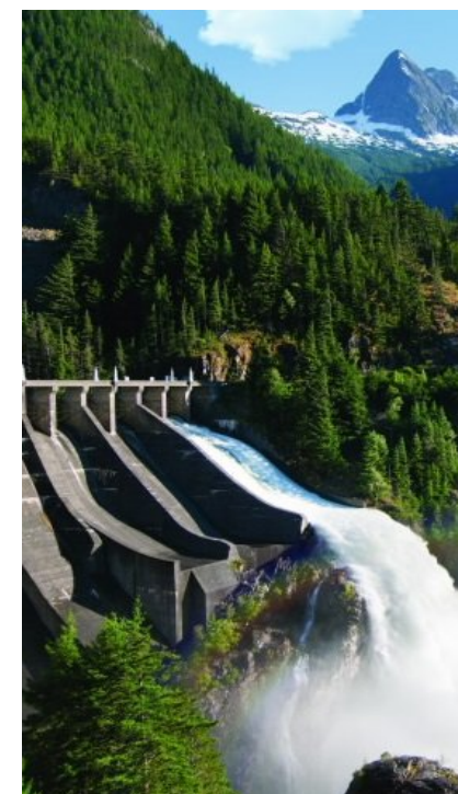
Hydroelectric Project Operations
