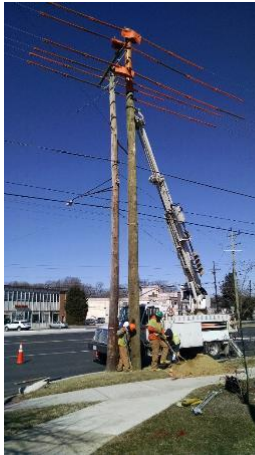
Figure 22: OSP Crew Replacing a Pole
