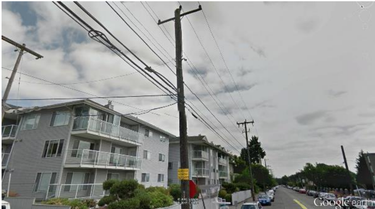
Figure 20: Example of a Pole in Seattle with Congested Communications Space (Google Earth)
