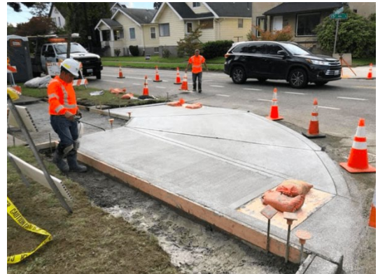
SDOT staff conducting sidewalk work in 2020. Source: SDOT.
