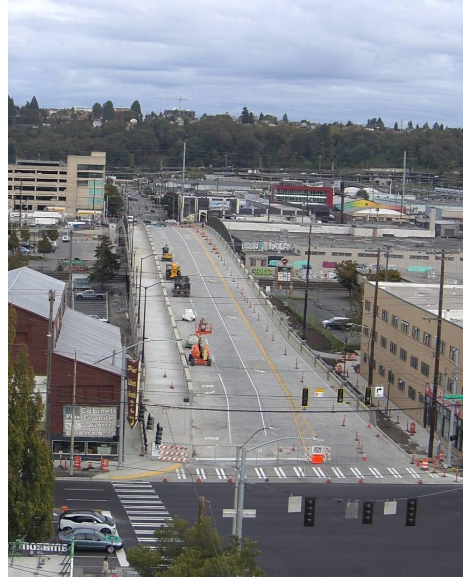
Lander St Bridge completed Oct 2020
