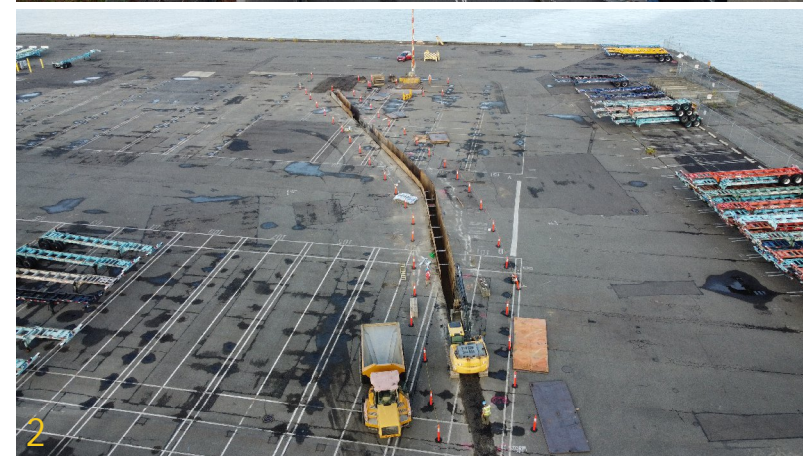
1. Sep 26, 2023: Ductbank alignment, looking south on Terminal 46
