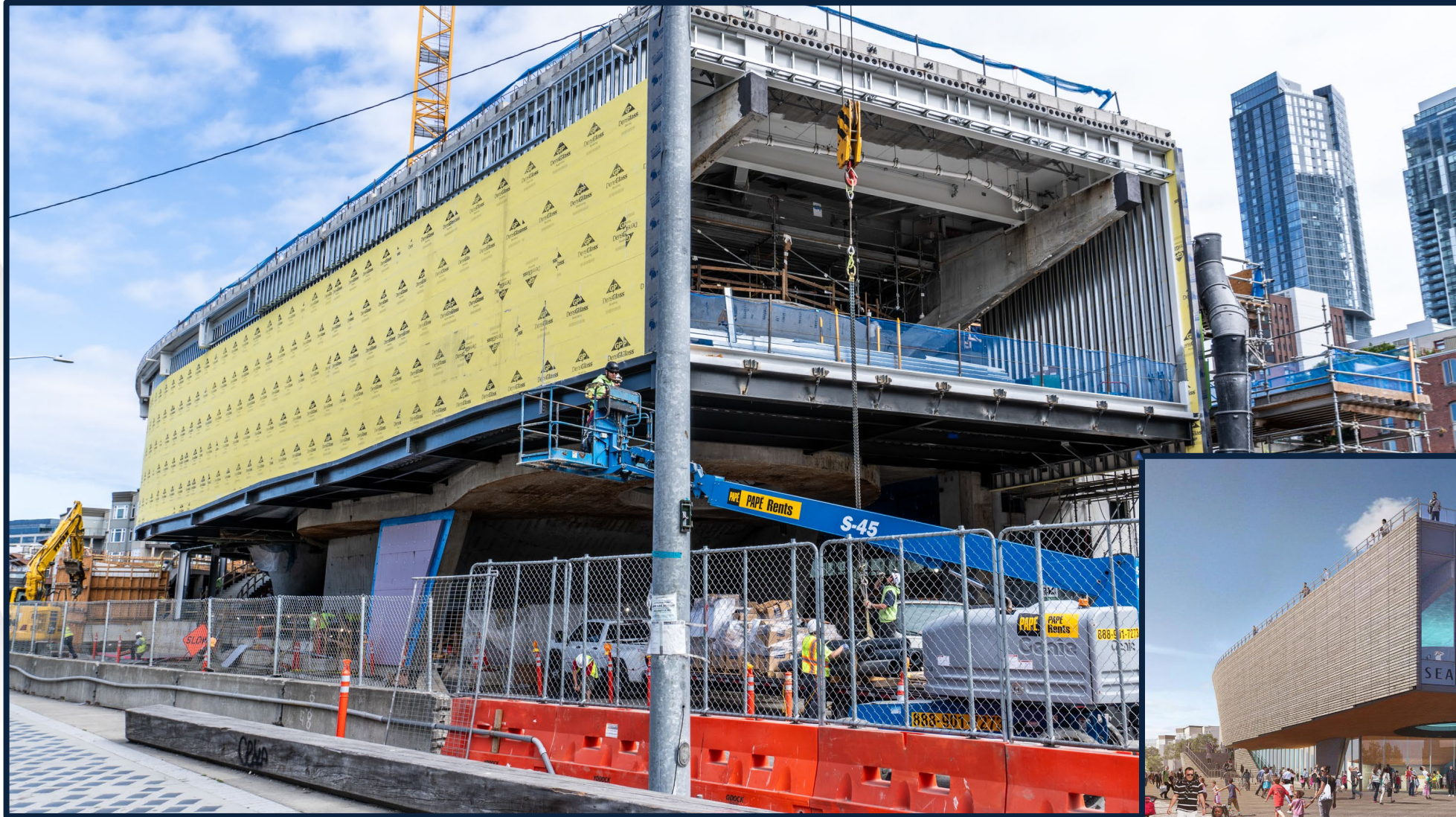
Ocean Pavilion view north
