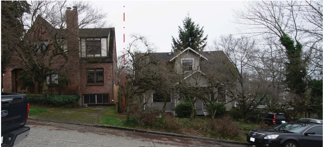
Figure 16: Site photo looking at northeast corner on NE 71 st St
