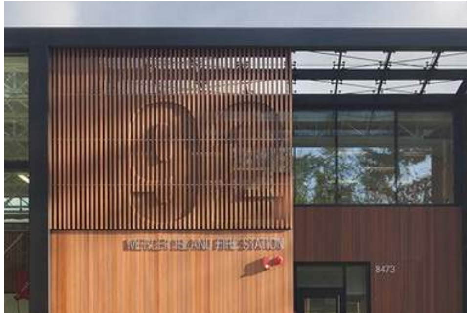
WARM-TONED WOOD AT FACADE - MERCER ISLAND FS 92 Miller Hull Partnership
