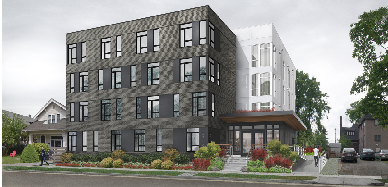
4710 20th Ave NE (Under Construction)
