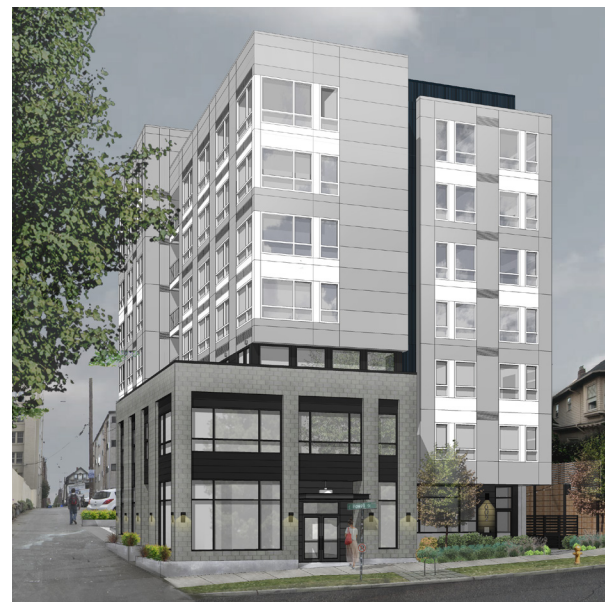
600 E Howell St (Under Construction)
