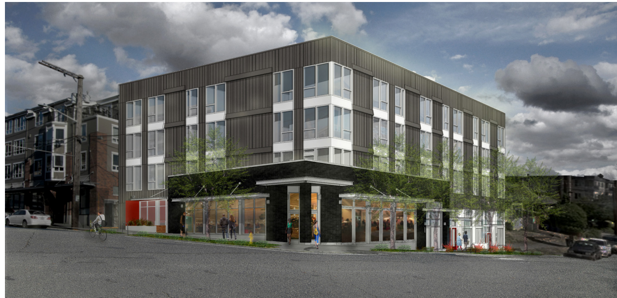
800 5th Ave N (Under Construction)
