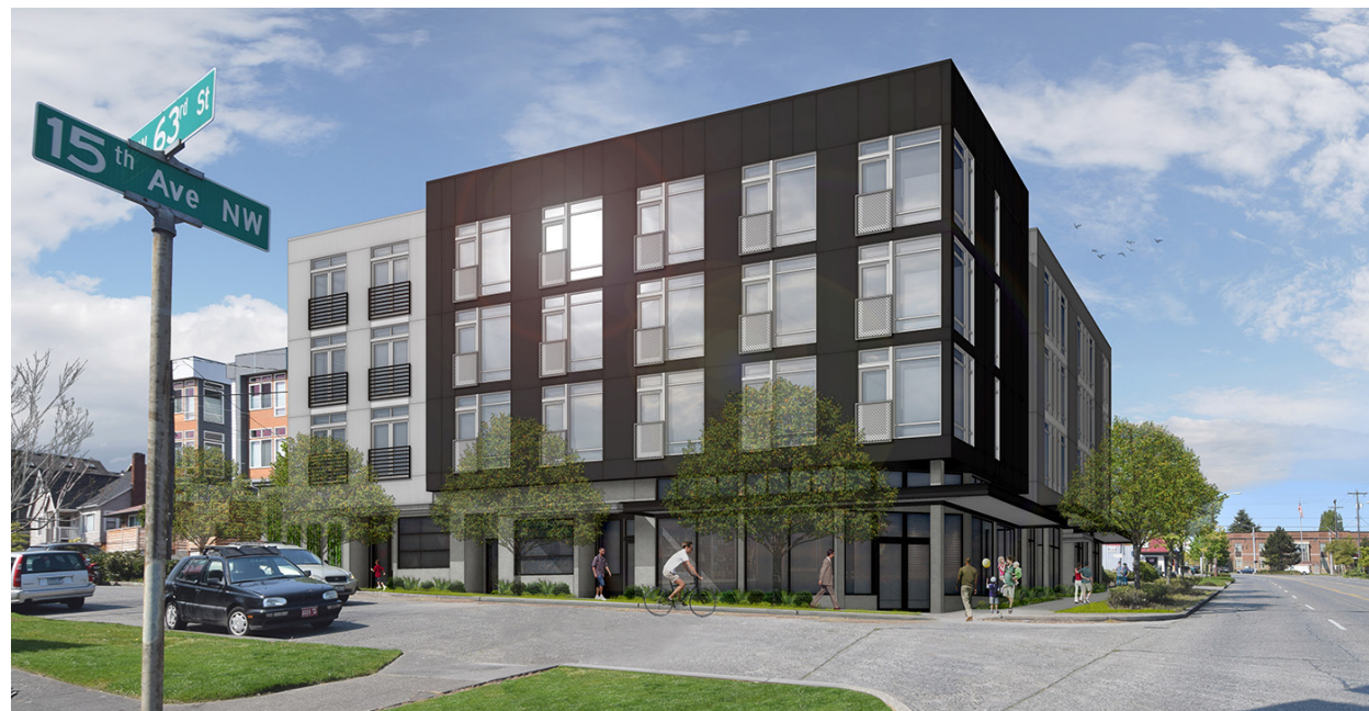
6301 15th Ave NW (Under Construction)
