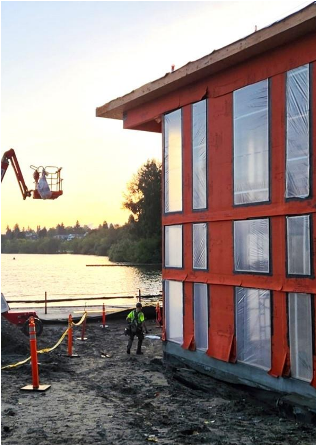
GREEN LAKE SMALL CRAFT CENTER, CONSTRUCTION 2023 SOURCE: COUNCILMEMBER STRAUSS NEWSLETTER
