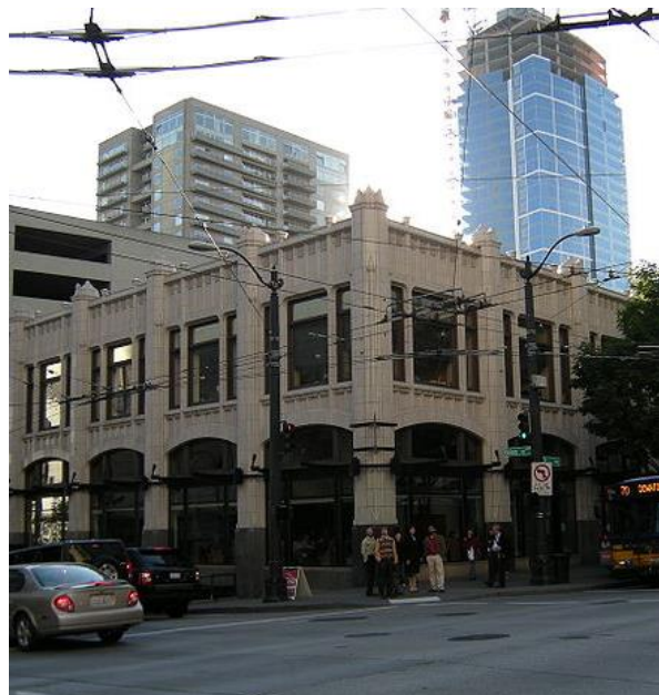
Figure 11 Picture of the Mann Building
