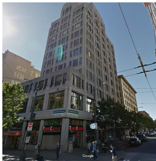
Figure 13 Picture of the Olympic Tower building
