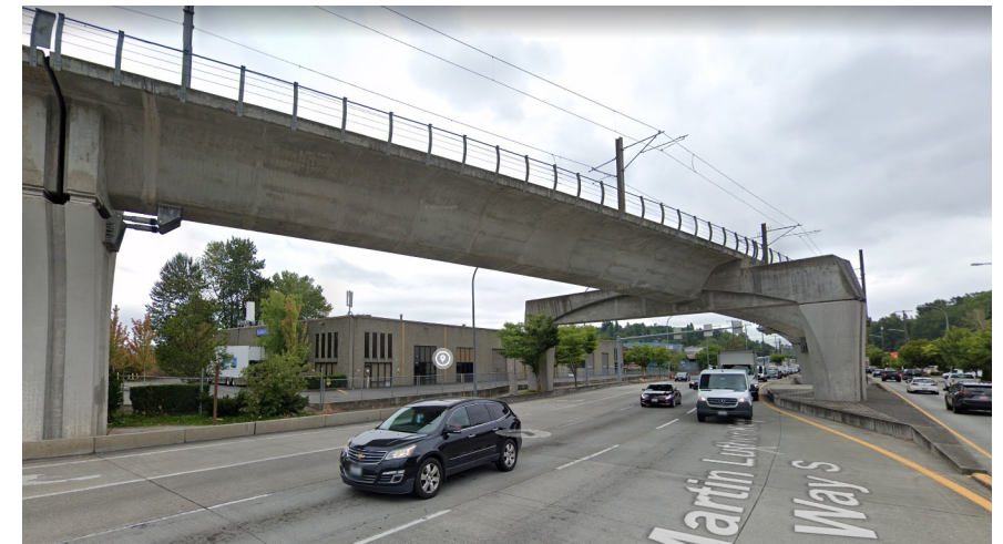
Google street views Lynnwood Link Extension (top) and Central Link on MLK Way (bottom) show how elevated structures can impede sightlines and obstruct center turn lanes. (Images: Google street view)
