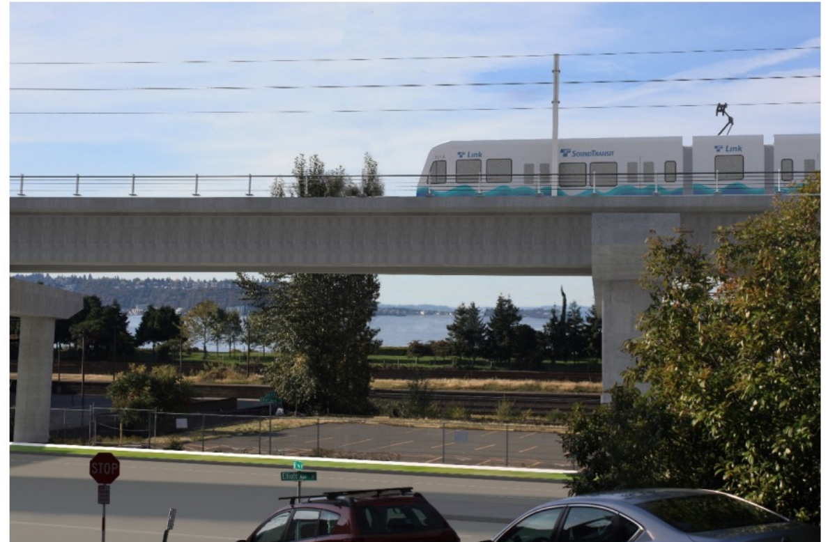
Rendering of SIB-1 along Elliott Avenue West. (Image: WSBLE DEIS Appendix N.2)
