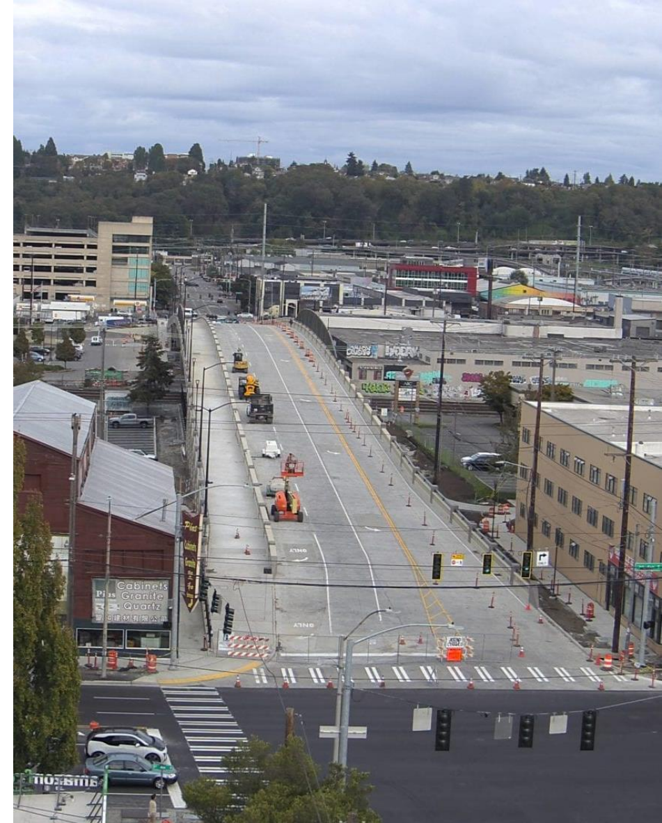
Lander St Bridge completed Oct 2020
