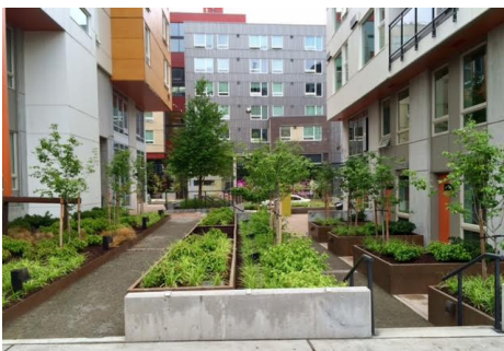
A mid-block pathway through a residential development is lined with unit entries, planters, and windows. A change in paving signifies the transition to semi-private space.
