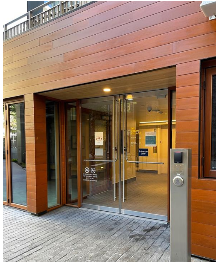
Elevator to Second Ave
