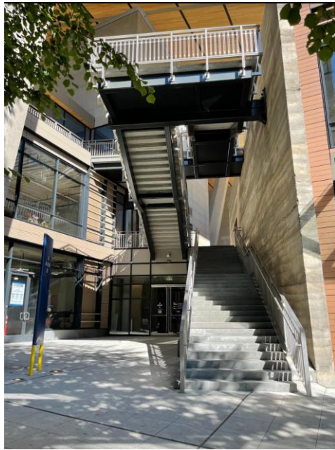
1st Ave. Promenade - Grand Staircase mid-block looking east showing building setbacks, public stair and seating.
