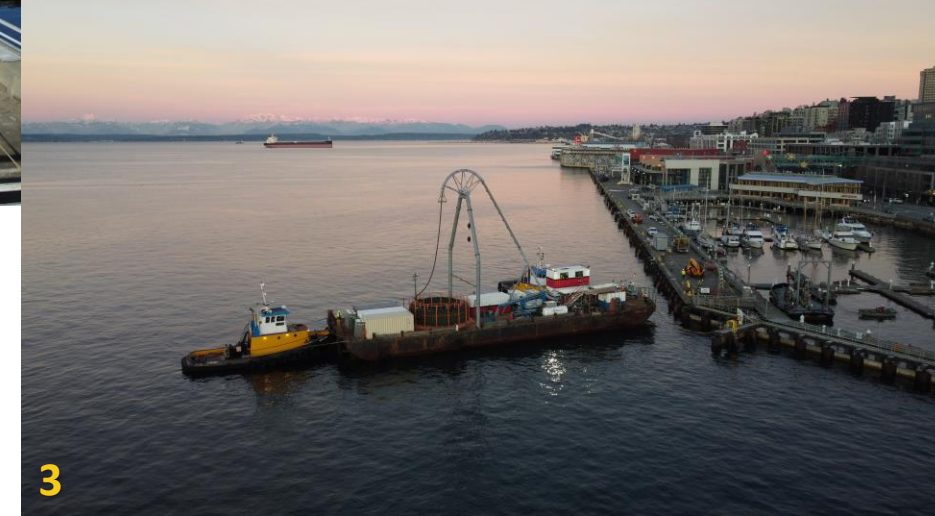
1. Jan 15, 2024: Submarine Cable pulling rig on Pier 66 2 and 3. Jan 15, 2024: Submarine Cable lay at Pier 66
