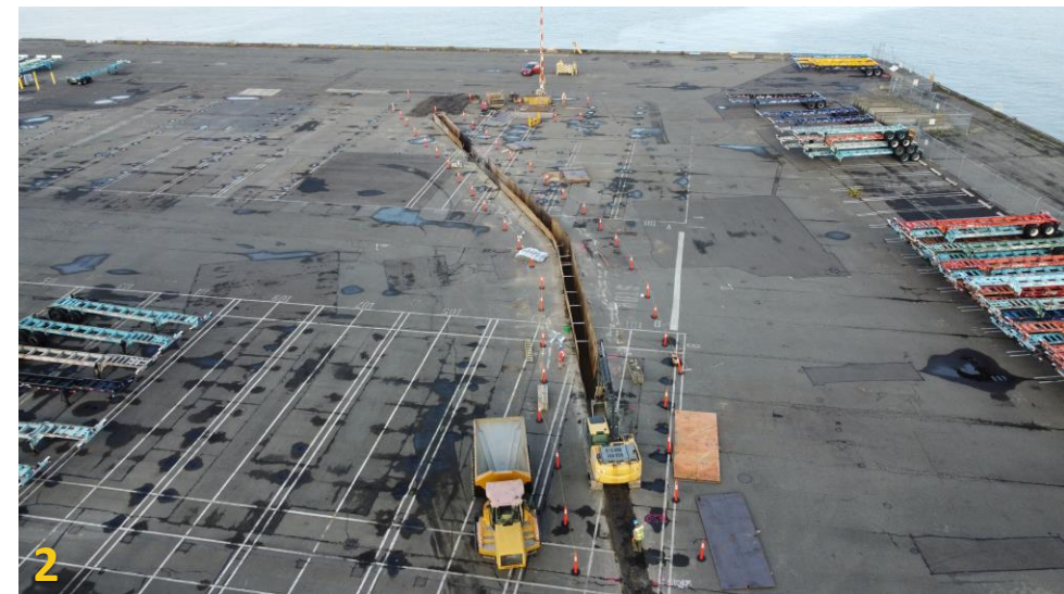
1. Sep 26, 2023: Ductbank alignment, looking south on Terminal 46
