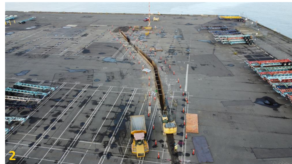
1. Sep 26, 2023: Ductbank alignment, looking south on Terminal 46
