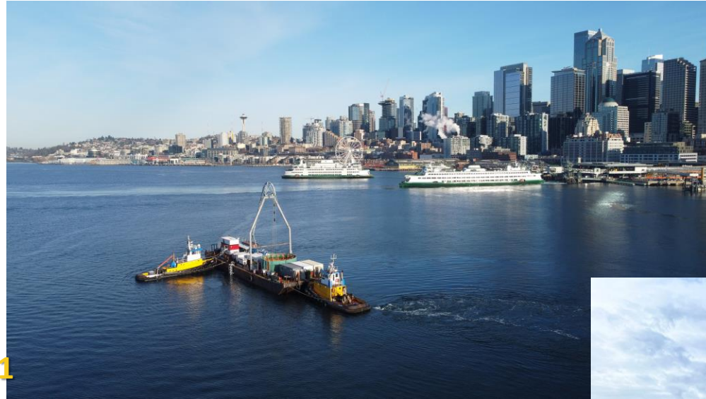
1. Jan 15, 2024: Submarine Cable lay
