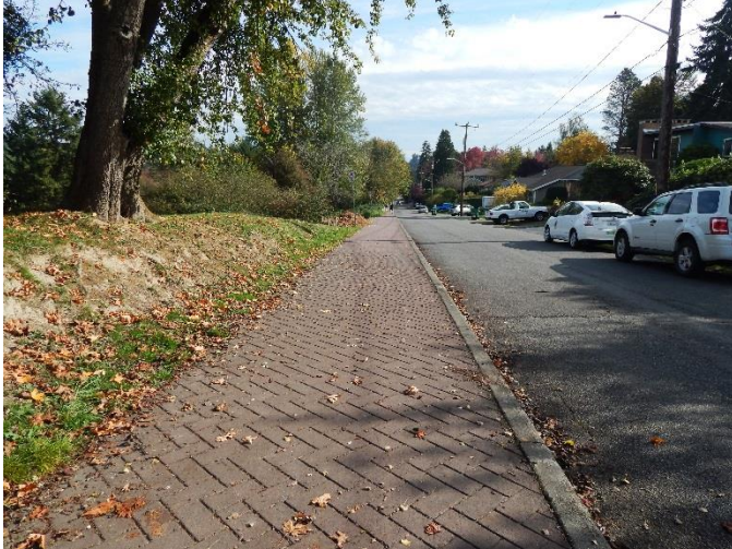
Grade-separated asphalt pathway
