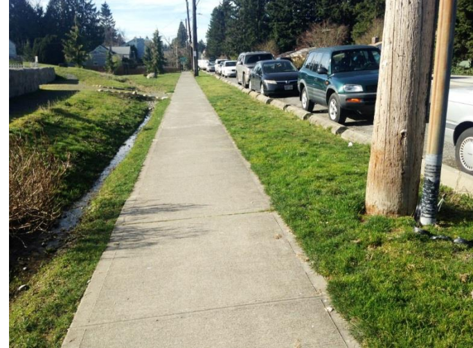
At-grade concrete pathway
