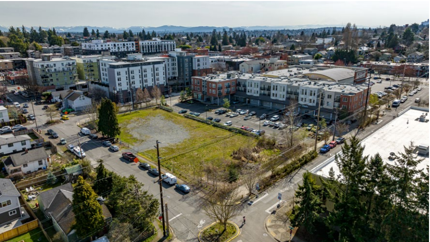
NW Corner Aerial View
