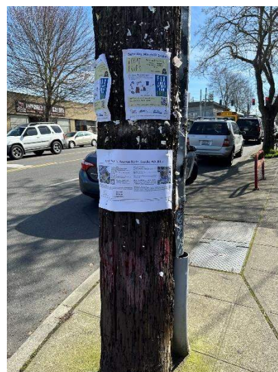
Telephone pole located at southwestern corner of intersection of Greenwood Avenue N and N 84 th St, facing sidewalk
