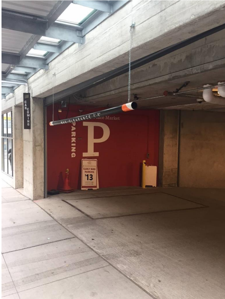
Parking Garage Entry Signage
