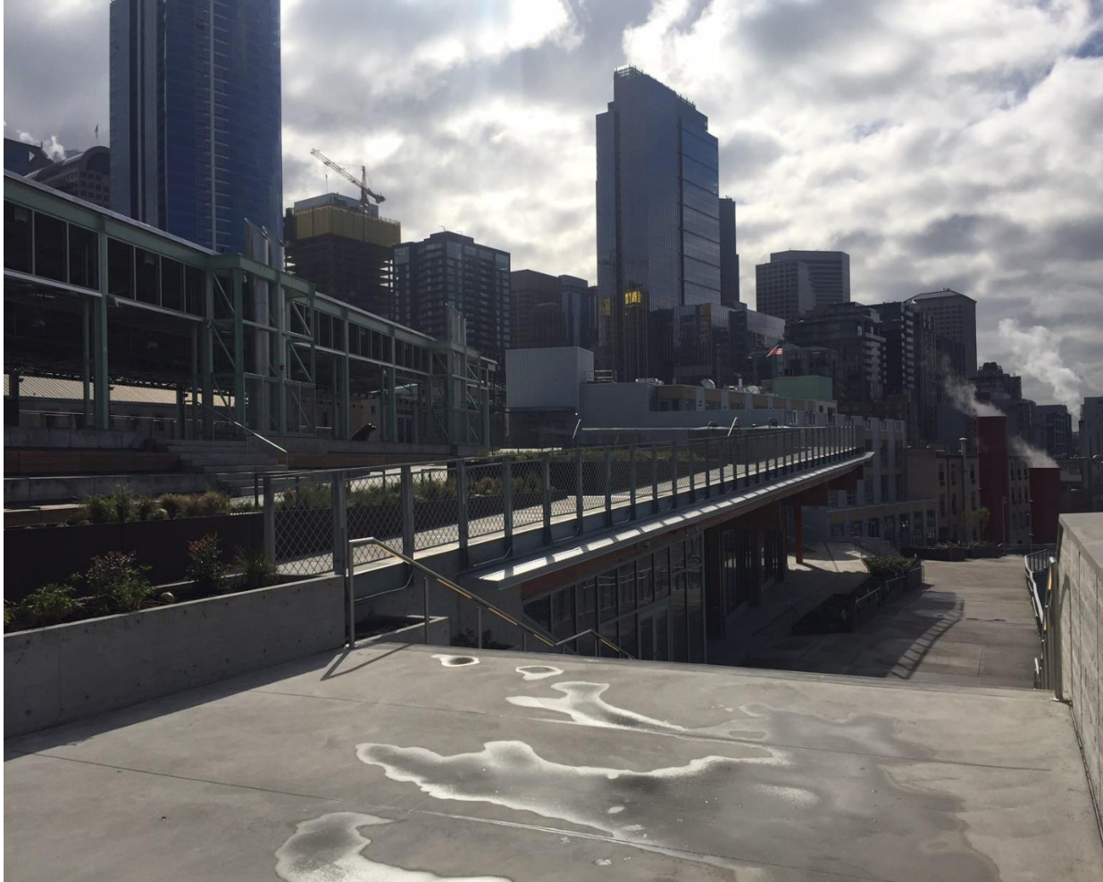
West Side – looking south
