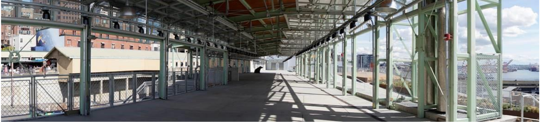
Covered Canopy Area – looking south
