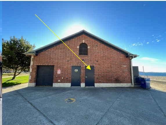
North End Storage Area
