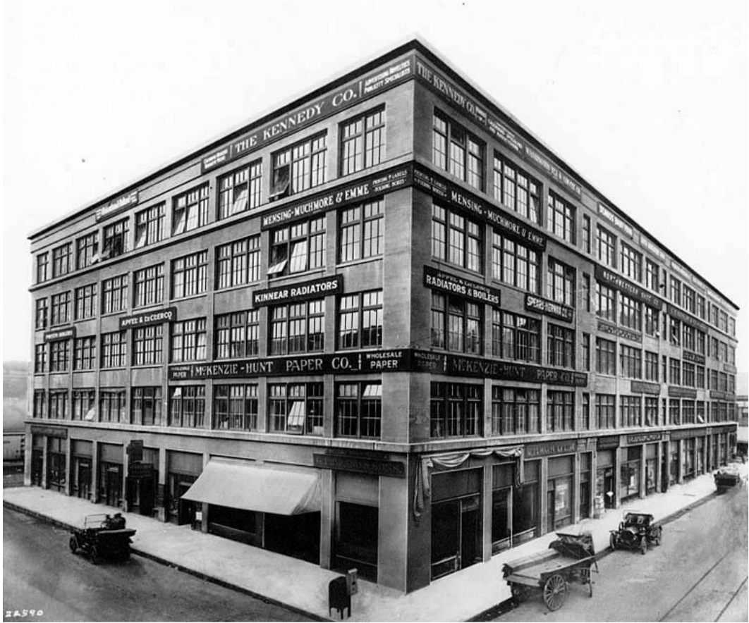
Maritime Building, 911 Western Avenue, 1911
