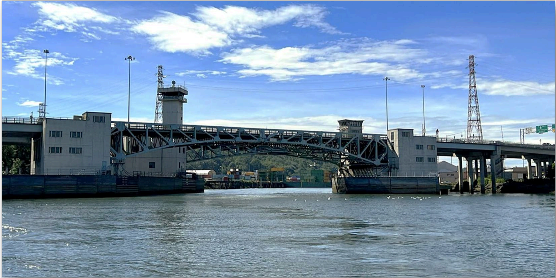
The northbound SR 99 First Avenue South Bridge links South Park and Georgetown across the Duwamish River.
