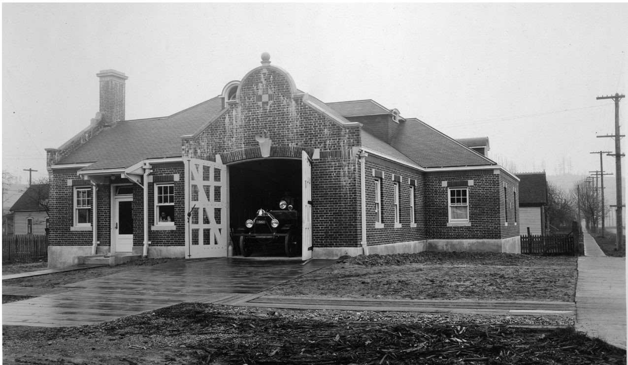
former Fire Station 26, 8201 10 th Avenue S, 1921
