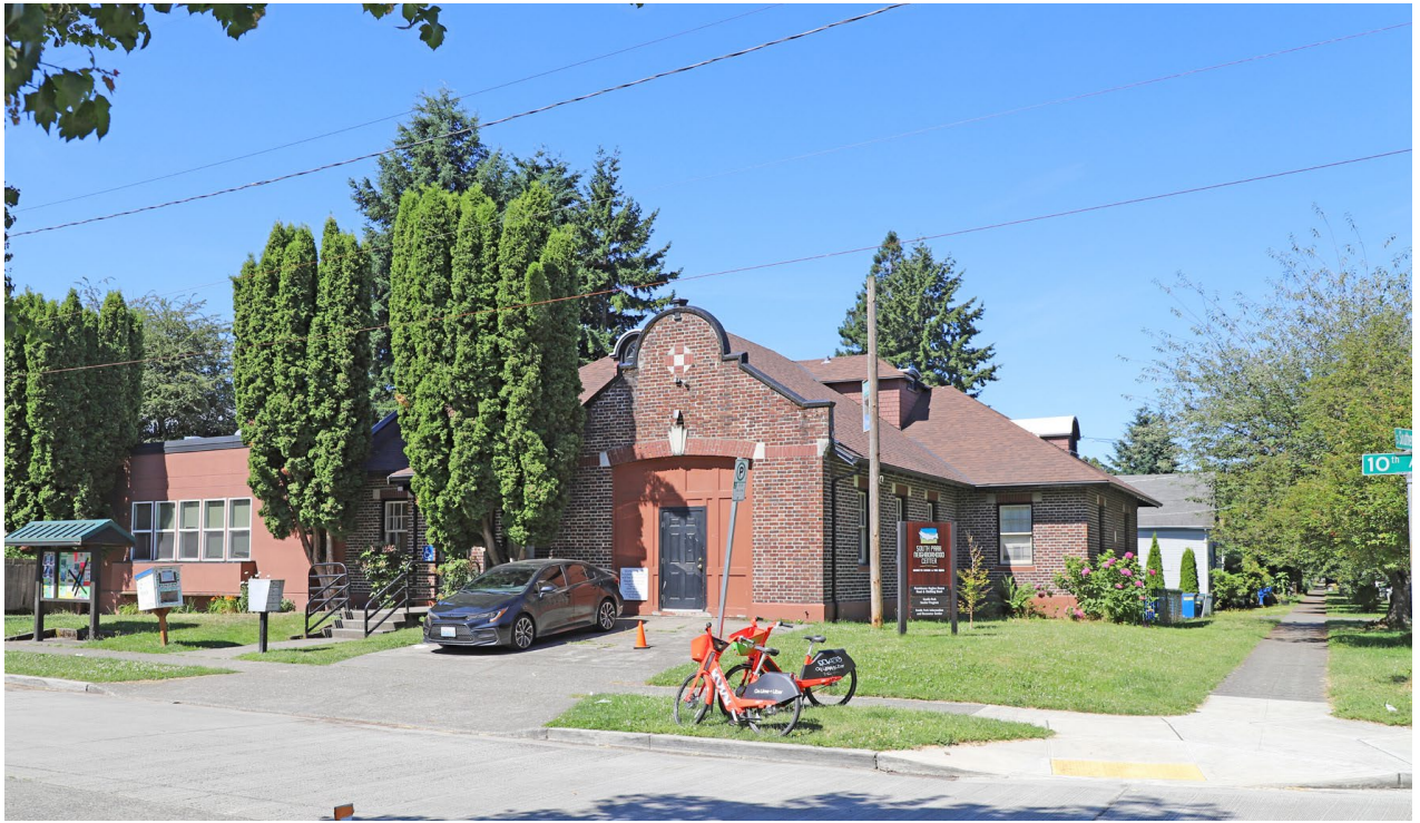
former Fire Station 26, 8201 10 th Avenue S, 2021
