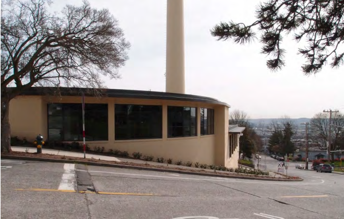
Yesler Terrace Steam Plant, current
