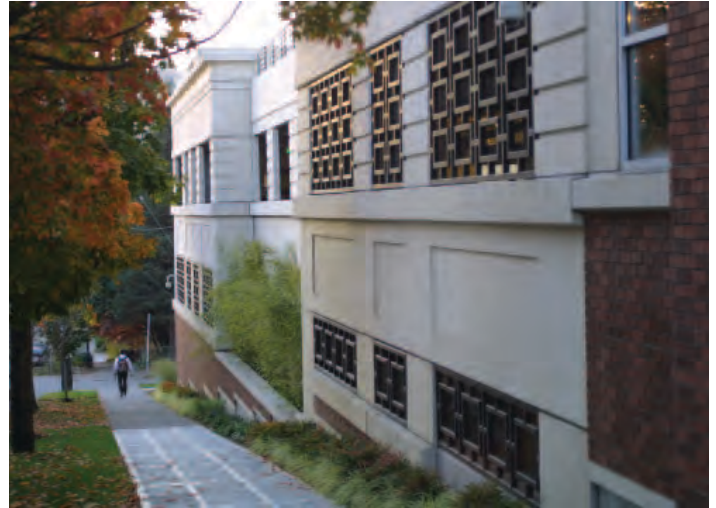
Street Frontage Architectural Features
