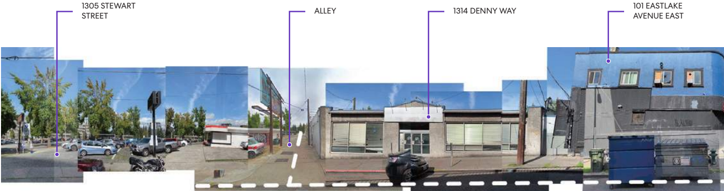
3. Lower Denny Way - Looking North at Project Site
