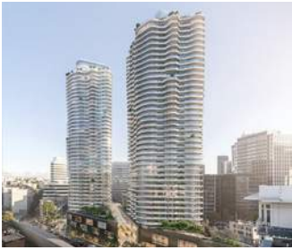
9. 1200 Stewart Street (Under Construction)
